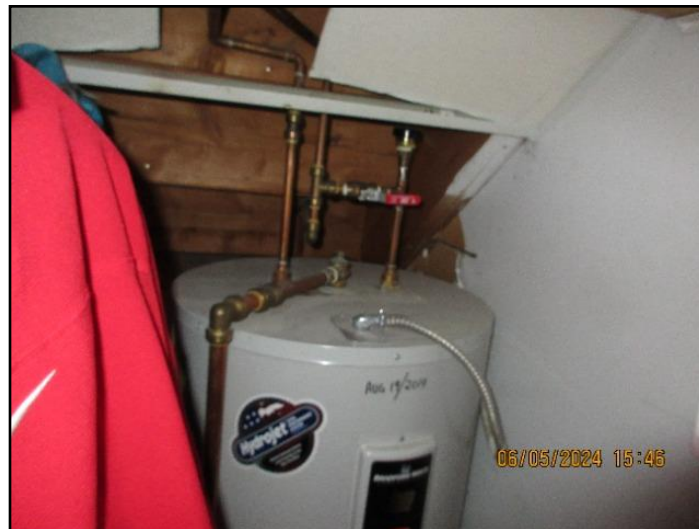
46. Utility room under stairs
