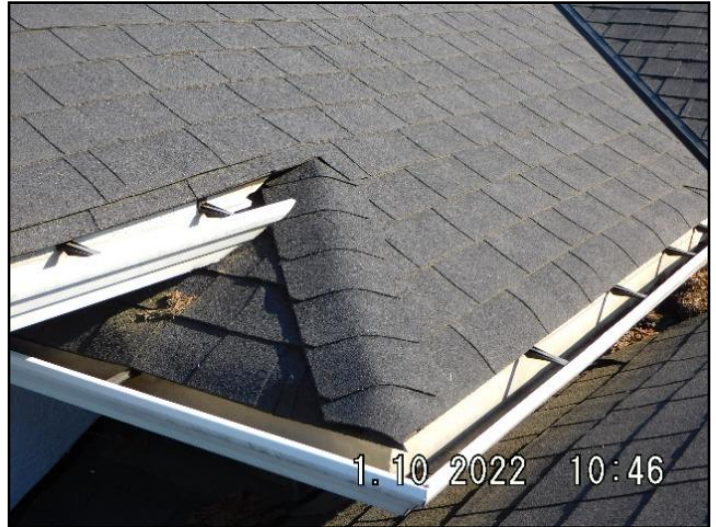
2. The inspection of the roofing system...
