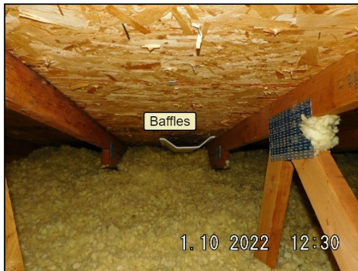
81. Roof and soffit vents
