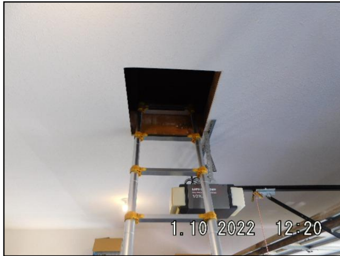
83. From access hatch
