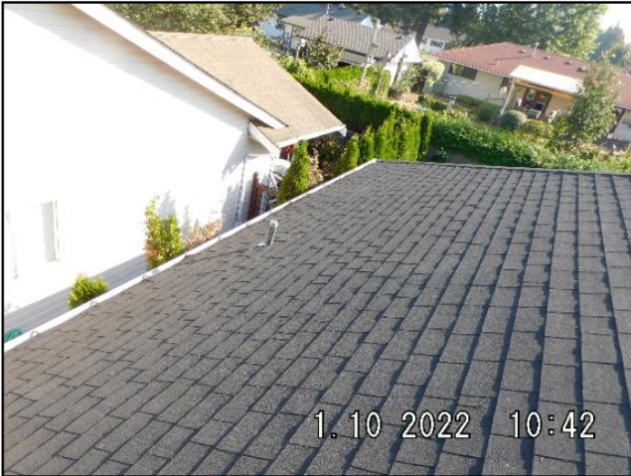
1. The inspection of the roofing system...
